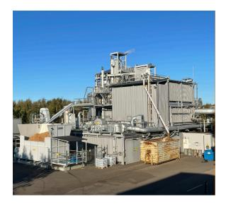
**EXPERTISE** A new innovative biomass gasification process. A new standard is reached with the Wood-Roll® process improving the thermal yield and syngas quality to levels never even imaginable before. There are two installations in Sweden today: a test plant of 0,5 MW and one industrial 6 MW WoodRoll®.
